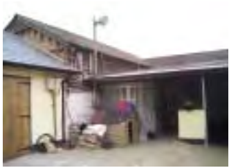
The old building before work.
