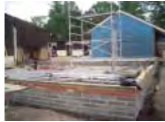
New foundations are put in
