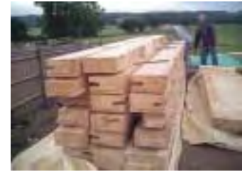
Timber frame arrives on site.
